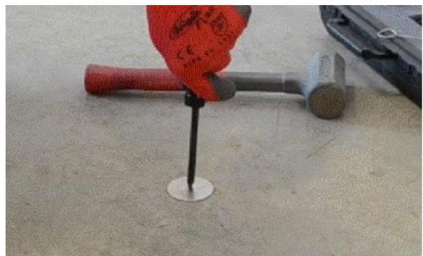
Figure 5. Tightening the Secured Cover
