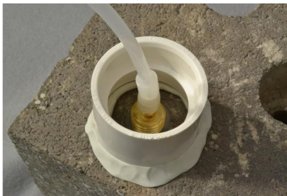
Figure 10. Water dam used for leak detection
