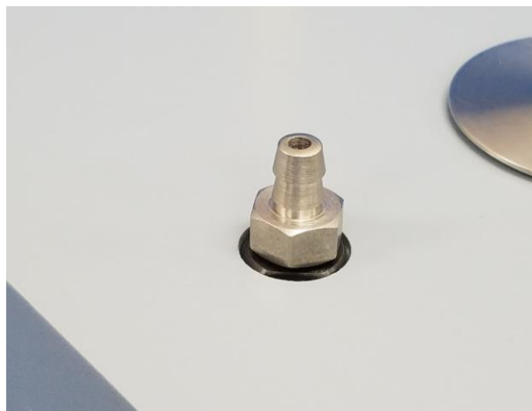
Figure 6. Mini Vapor Pin® Sampling Device Installation Complete
